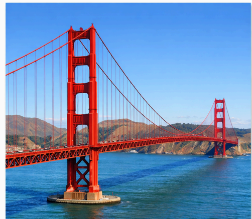
Golden Gate Bridge (San Francisco)
